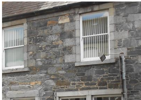
Unpainted coursed rubble whinstone with granite window margins and sills
