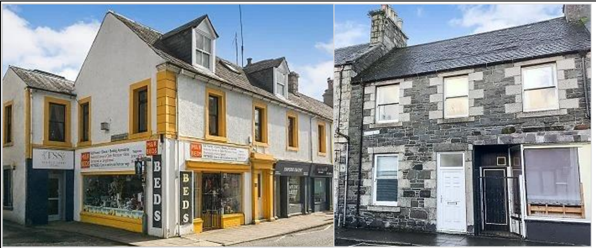
Shop on Morton's entry with front and side windows, some oversized fascia signs. Shop on Albert Street - simple style in a simple building.
