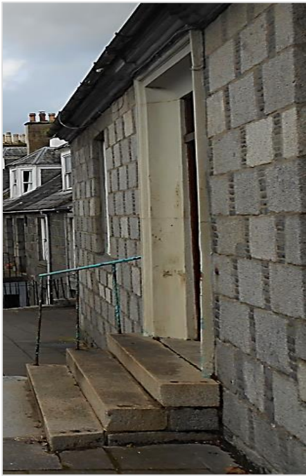
Granite blocks in distinctive coursing with mouse ladder snecking stones in vertical spaces between blocks
