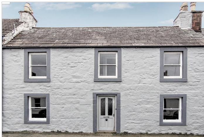
Vernacular, 2-storey, 3-bay terrace on Creebridge.
