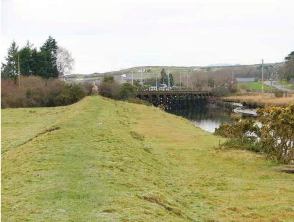
PHOTO 1: TYPICAL EXAMPLE OF AN EMBANKMENT
