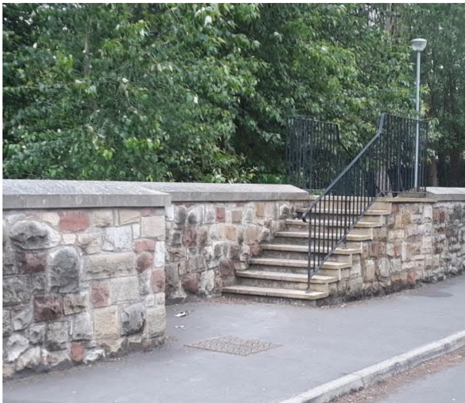
PHOTO 4: TYPICAL EXAMPLE OF ACCESS POINT WITHIN A FLOOD WALL
