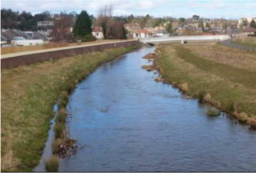
PHOTO 2: TYPICAL EXAMPLE OF BRICK FACED WALL
